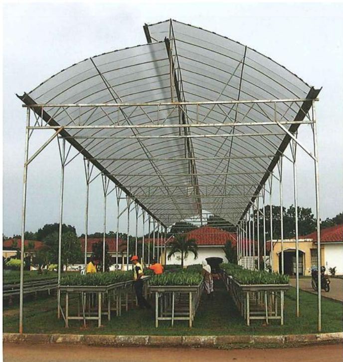
Plant house BX-1 system A
